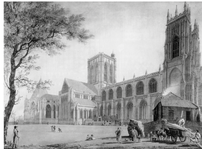
Drawing by James Malton in 1794, showing the newly revealed north side of the Minster following the demolition of medieval buildings
