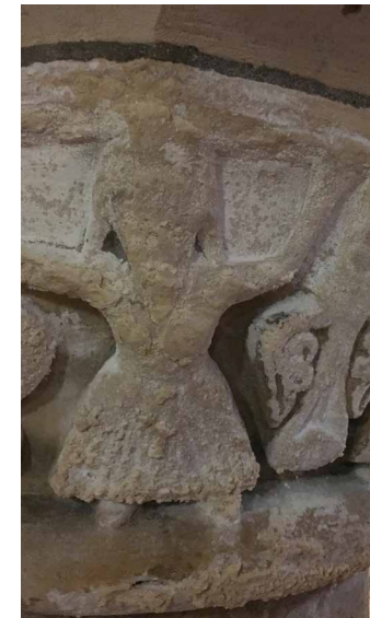
Stone corrosion
